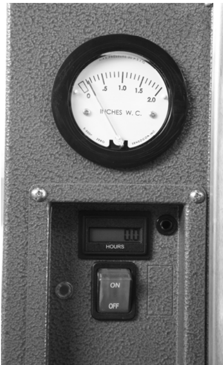
Module Control Panel
